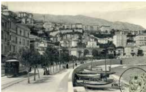
Vers 1905. Le boulevard de la Condamine devenu Albert I er . Around 1905. The Condamine Boulevard which later became Albert I er .
